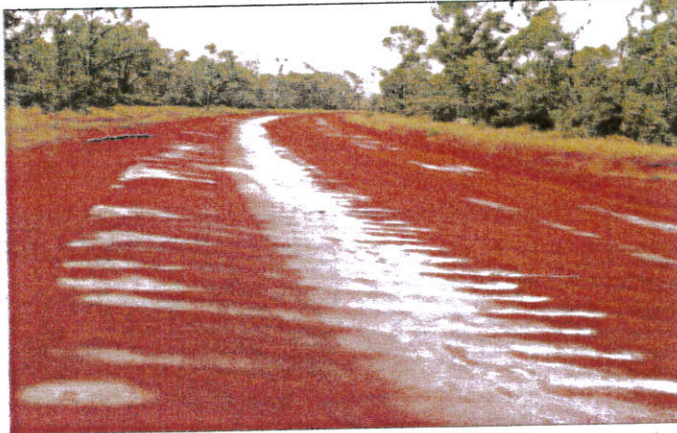
The Northern Australia Roads Program will deliver up to $223.8 million for projects in Queensland, with $37.3 million to be provided in 2017-18.
