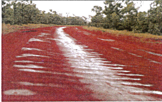
The Northern Australia Roads Program will deliver up to $223.8 million for projects in Queensland, with $37.3 million to be provided in 2017-18.
